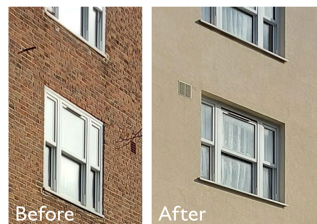
Before After Example of external insulation
