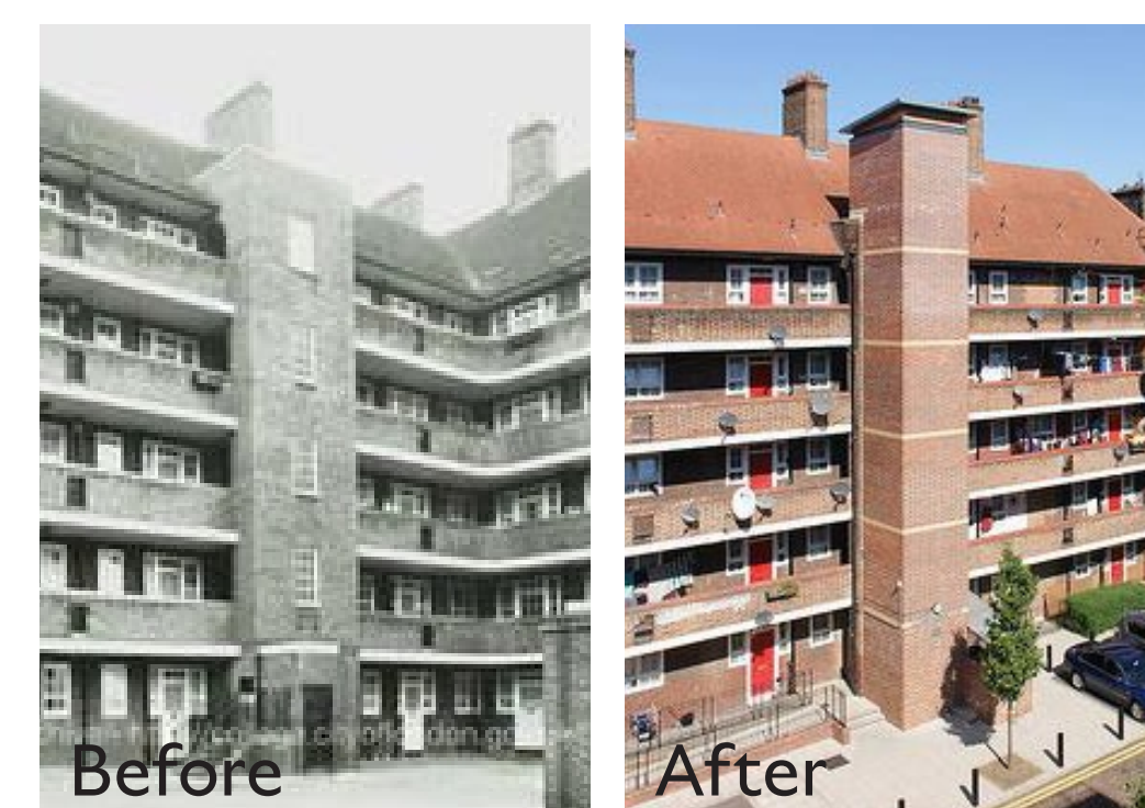
Before After Example of new lift
