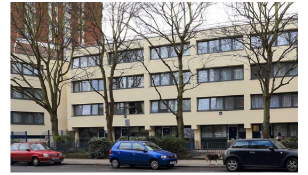
Example of external insulation added to Denton Estate in Camden
