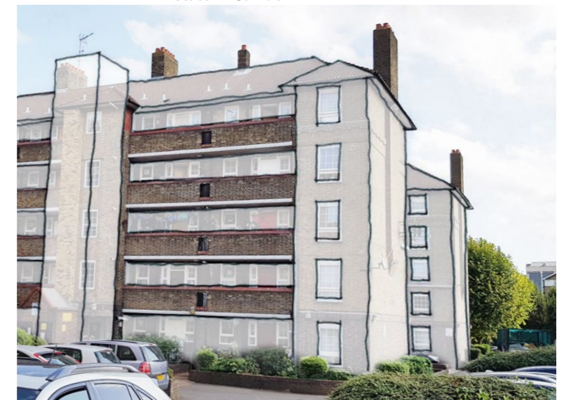
Proposed example view of Montrose House with layer of insulation on the outside to keep homes warm.
